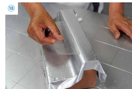
Adjust the film with a spatula to release water and air bubbles that appear on the surface, being careful to smooth corners. Finish by wiping away excess water with a cloth.
