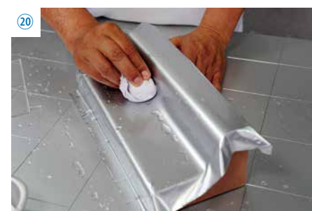
Adjust the film with a spatula to release water and air bubbles that appear on the surface, being careful to smooth corners. Finish by wiping away excess water with a cloth.
