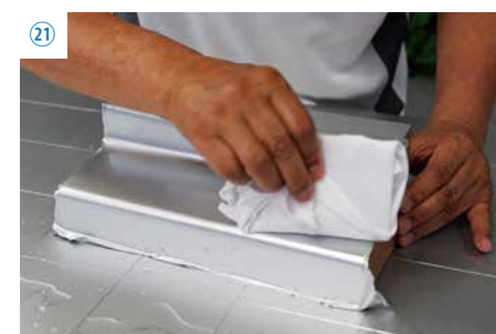
Adjust the film with a spatula to release water and air bubbles that appear on the surface, being careful to smooth corners. Finish by wiping away excess water with a cloth.
