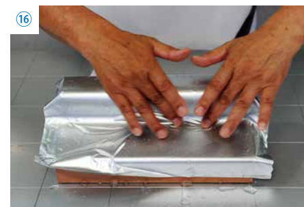
Adjust the film with a spatula to release water and air bubbles that appear on the surface, being careful to smooth corners. Finish by wiping away excess water with a cloth.
