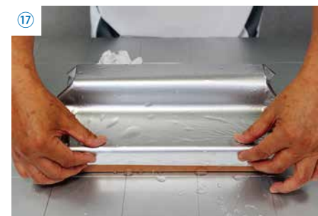
Adjust the film with a spatula to release water and air bubbles that appear on the surface, being careful to smooth corners. Finish by wiping away excess water with a cloth.
