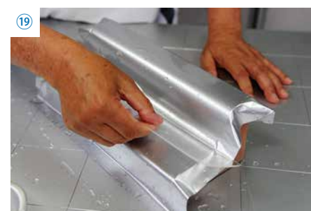
Adjust the film with a spatula to release water and air bubbles that appear on the surface, being careful to smooth corners. Finish by wiping away excess water with a cloth.
