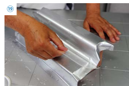
16 Adjust the film with a spatula to release water and air bubbles that appear on the surface, being careful to smooth corners. Finish by wiping away excess water with a cloth.
