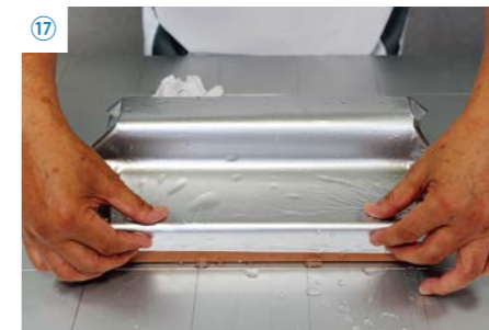
16 Adjust the film with a spatula to release water and air bubbles that appear on the surface, being careful to smooth corners. Finish by wiping away excess water with a cloth.
