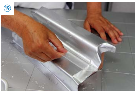
16 Adjust the film position, releasing of water and foam generated in the surface and clearance corner with a rubber spatula or squeegee, then it adhere to the surface and wipe away the water with a cloth.
