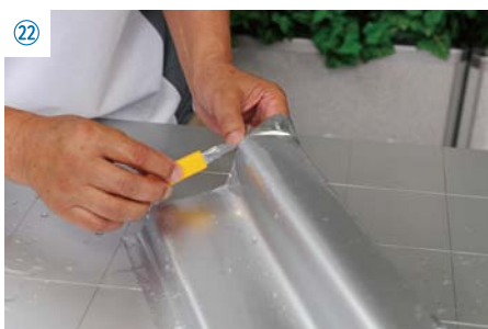
22 Cut out the extra edge carefully while wet with water. When the film is dried up, it becomes adheres to the surfaces between the film and paste. It is very difficult to cut out the film.
